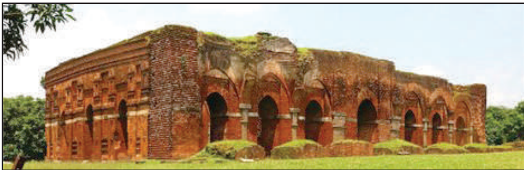
Darasbari Mosque of Chapainawabganj
